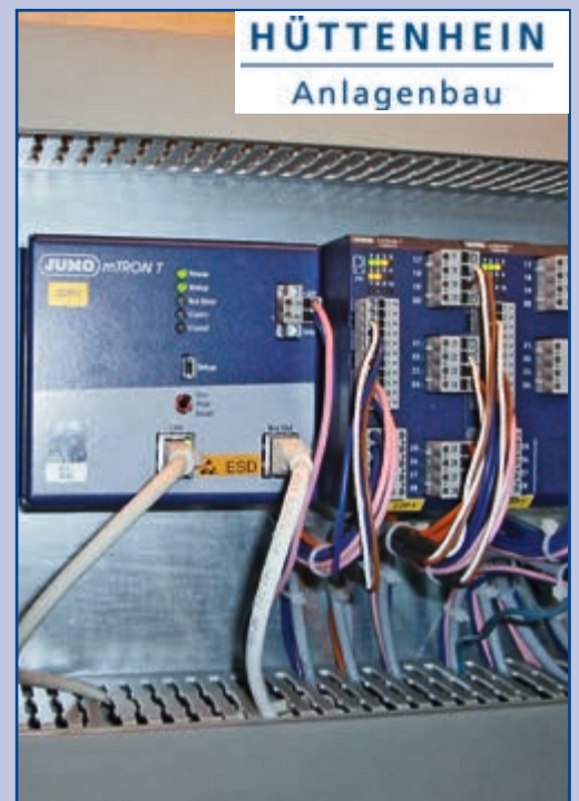
Installation situation of the JUMO mTRON T
